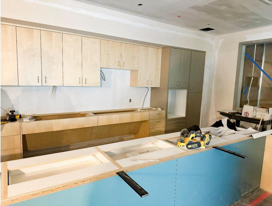
Things are taking shape! Kitchen cabinets being installed in the kitchen.
