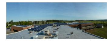
*Solar Panels:* 1,200 solar panels that will generate over 300 MWh of electricity per year, enough to
